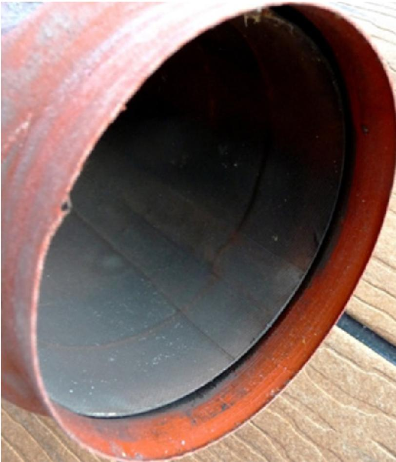
**Contaminated Air Duct. Quelle: AERO**
